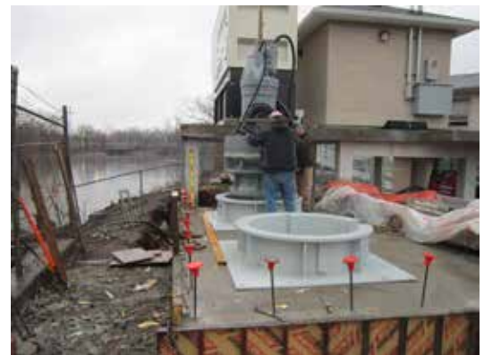
Patrick Carberry, PE to supervise the pump installation
